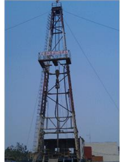
Image: Drilling a geothermal well in 2012 at the Procter & Gamble plant in Xiqing China Source: Procter & Gamble
