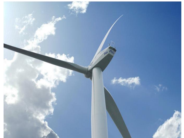
Image: Procter & Gamble wind mill installed at the Coevorden plant in the Netherlands
